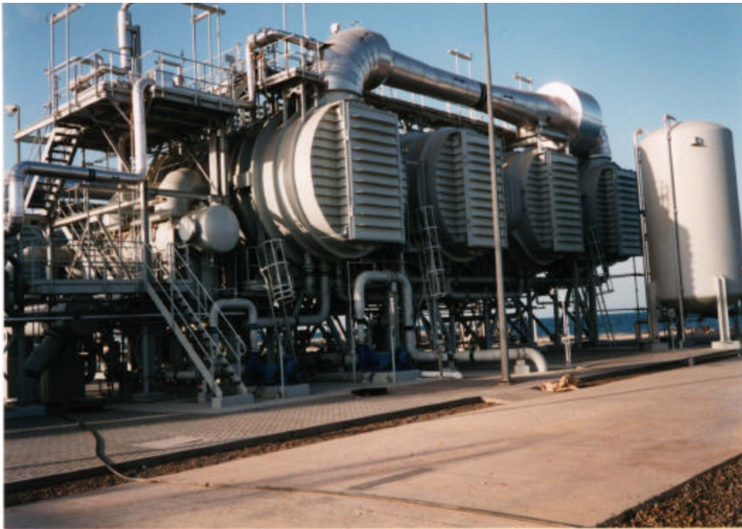
Figure 3.22 5000 M3/day 4 - Effect Thermo Vapour Compression. (Sidem Ltd)
