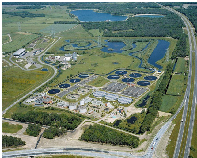
Figure 13.2 Overview of the STP Tilburg.
