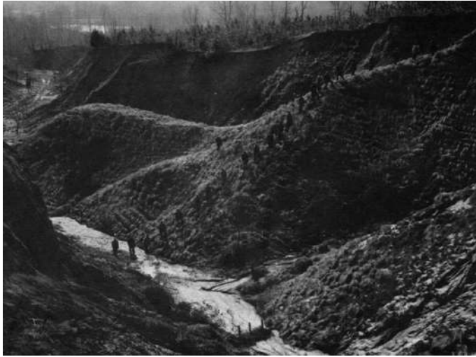
FIGURE 20.3 The YLT project reforested the most badly gullied land. In the case illustrated, strips of weeping lovegrass ( Eragrostis curvula ) were established to stabilize the actively eroding sandy gully sidewalls, and in the following winter, loblolly pine ( Pinus taeda ) seedlings were transplanted. Brush dams were constructed to stabilize thalweg areas before tree planting. (From Williston, H.L., The Yazoo–Little Tallahatchie Flood Prevention Project. A history of the Forest Service’s role. U.S. Forest Service. Southern Forest Experiment Station. Forestry Report R8-FR 8, pp. 63, 1988; Duffy, P.D. and Ursic, S.J. Land Use Policy , 8, 196–205, 1991.)
