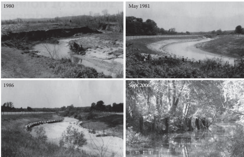
FIGURE 20.8 Vegetative streambank stabilization studies in Goodwin Creek proved successful, though expensive (From Bowie, A.J. Transactions of the ASAE , 25, 1601–1606, 1982; Bowie, A.J. Use of vegetation to stabilize eroding streambanks. U.S. Department of Agriculture, Conservation Research Report. 43, 24, 1995.) and stable reaches have survived without maintenance for more than 20 years. Prior to construction, banks averaged 3.2 m in height and channel bottom widths ranged from 9 to 12 m. The bed gradient is 0.0049, and the catchment area above the study reach is approximately 14 km 2 .
