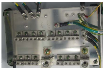
Large AC and DC ground bar for EGCs and GEC
