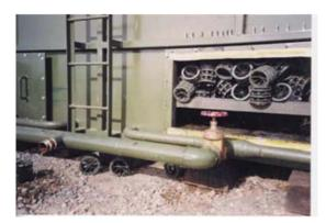
Figure 4.- Right: Support media used in SAF processes used (average diameter: 12-15 cm). Left SAF unit filled with Pall-rings type bulk material (average diameter 9 cm).
