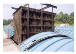
Figure 3.- Rope fixed support Ringlace. Clean (left); colonized by biofilm (right)
