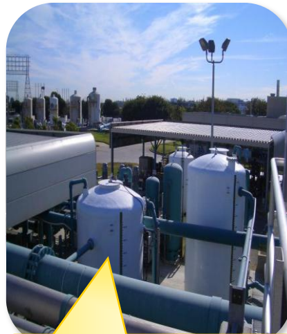
Coagulant Tanks
