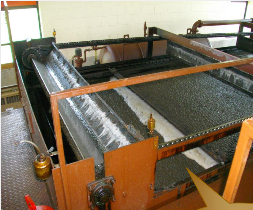
Sludge Thickeners
