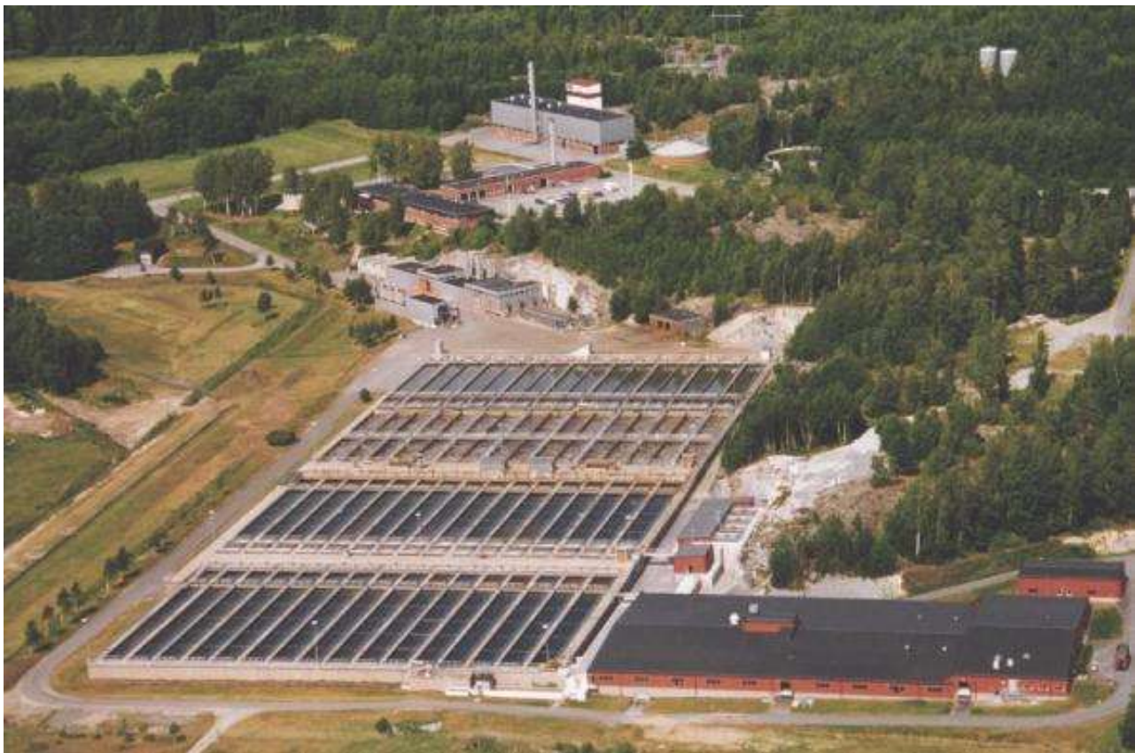
Himmerfjärden Wastewater Treatment Plant
