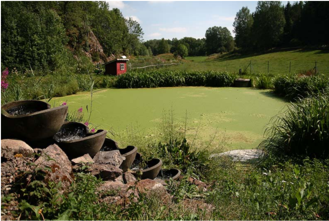
Flowforms in treatment pond in Norway
