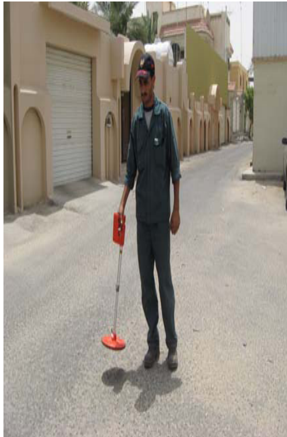
Locating Missing Valve
