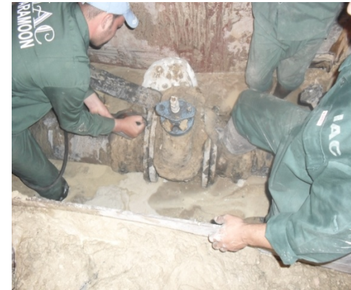
Replacement of Defected Valve
