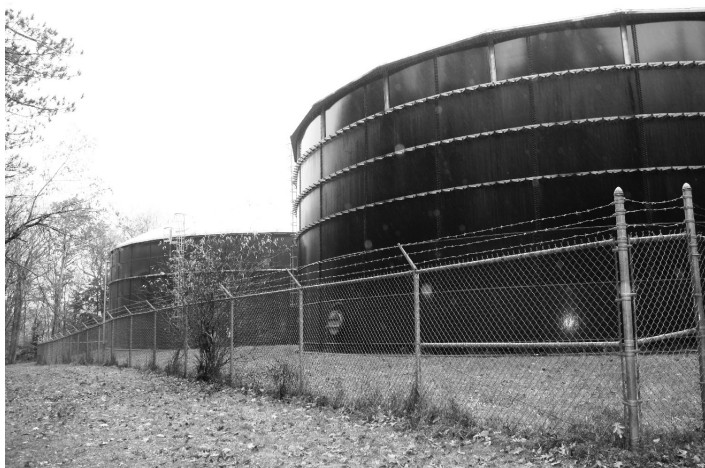
Figure 9.3 City of Oneonta water storage tanks.
