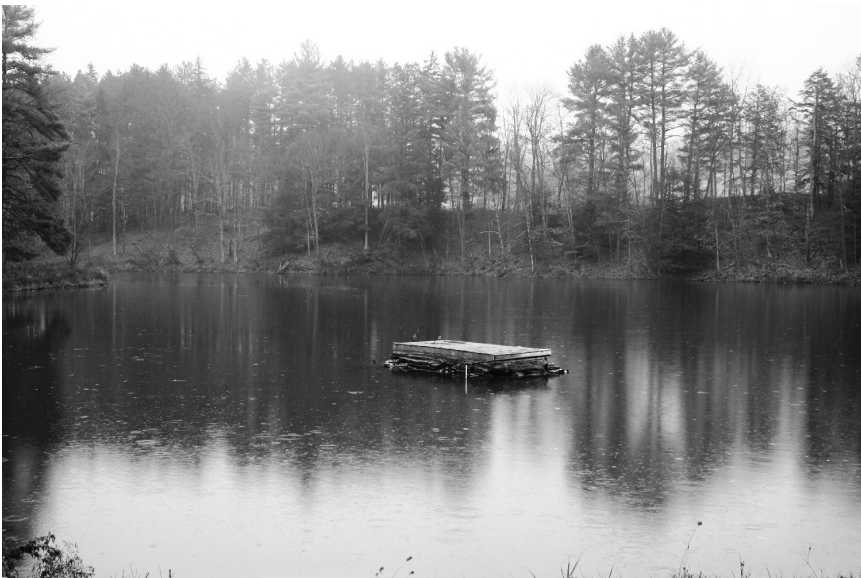
Figure 4.4 City of Oneonta lower reservoir (intake out of service).
