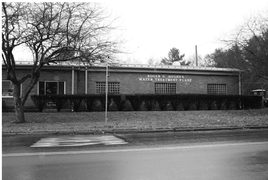
Figure 2.1 City of Oneonta, New York, water treatment plant.
