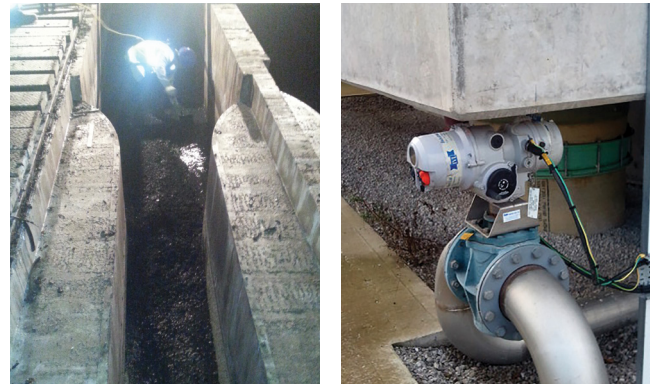
Figure 2.2 A large flume influenced by poor maintenance procedures allowing grit build up
