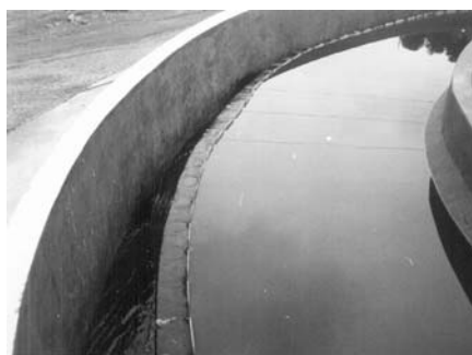
Figure 5.19. Effluent collection device (plate with V-notch weirs)
