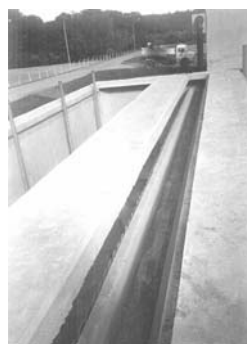
Figure 5.6. Effluent collection launder on the top of an anaerobic filter (Ipatinga WWTP, COPASA, Brazil)
