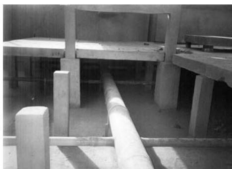
Figure 5.5. Sewage distribution device at the bottom of an anaerobic filter (Ipatinga WWTP, COPASA, Brazil)
