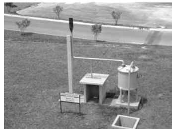
Figure 5.21. View of a hydric seal and gas burner (source: Ipatinga WWTP, Minas Gerais, Brazil)
