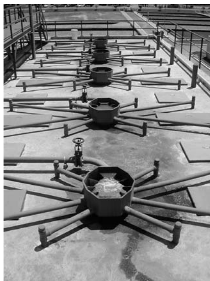
Figure 5.17. Influent distribution structure in a rectangular reactor (source: Ipatinga WWTP, COPASA, Brazil)
