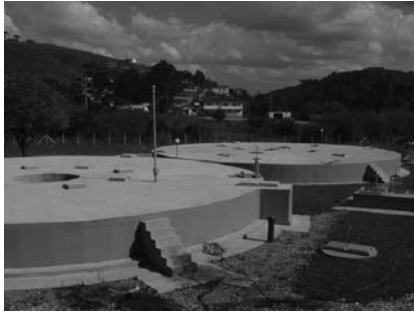
Figure 5.3. Anaerobic filter after upflow anaerobic sludge blanket (UASB) reactor (source: Colombo WWTP, SANEPAR/ Brazil)
