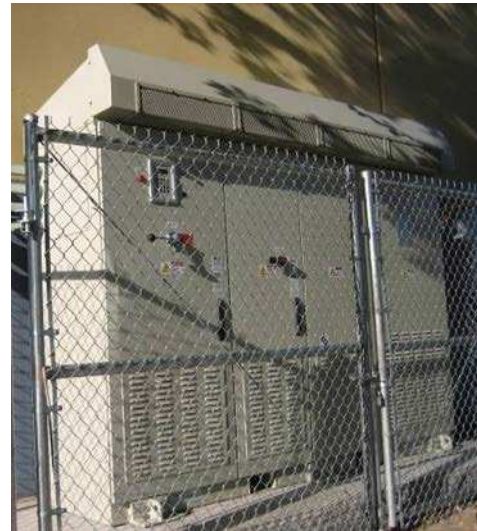
Figure 34: Central Inverters Are Used in Medium to Large Commercial Installations
