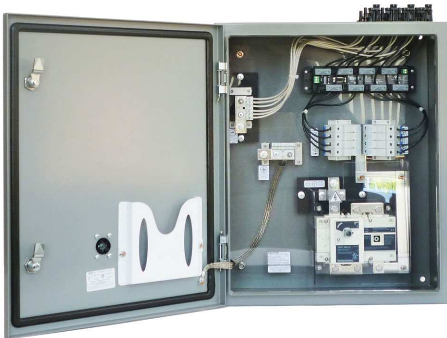
Figure 52: Combiner Box (courtesy of Solar Professional Magazine)
