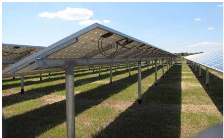
Figure 38: Ground-Mounted PV Arrays Often Use a Combination of Pole and Racking Designs for Simplicity
