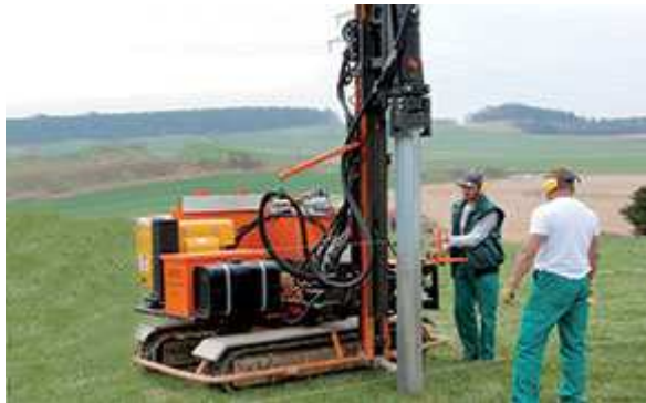
Figure 43: Foundations for PV Array Structures May Use Driven Piles or Anchors (Source: Schletter)
