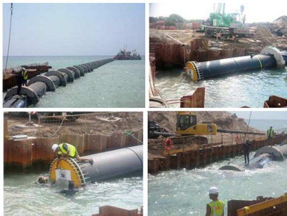
Figure 9: Installation of outfall for Llobregat desalination Plant (47.5 MGD) Spain (Pankratz 2009)
