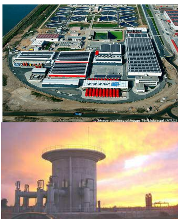
Figure 11: An aerial photograph (left) and WWTP Equilibrium Tower (right) of the Barcelona Desalination Plant
