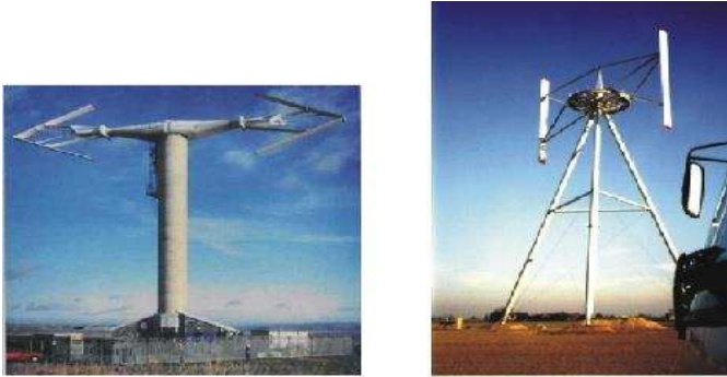
Figure 4: To the left is an H-rotor developed in the U.K. and to the right is one of the Heidelberg rotors.
