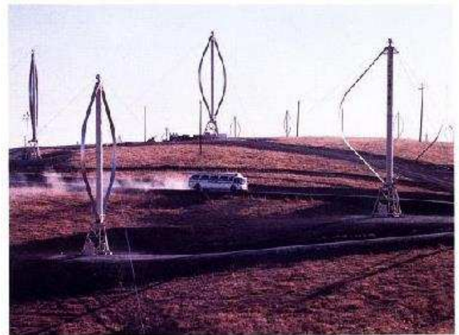
Figure 3: A Flow wind farm
