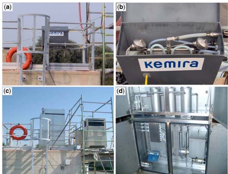
Figure 54 The first PFA hyproform production system (kemira Oyj) used in full-scale studies: prototype (a, b – 2005) and pilot system (c, d – 2006).
