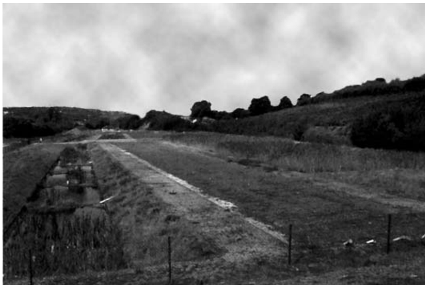
Figure 8.4. Constructed wetlands for treating AMD from the former Wheal Jane mine in Cornwall, south-west England. Aerobic, anaerobic (buried) wetlands and a rock filter system are shown, in sequence, from right to left.
