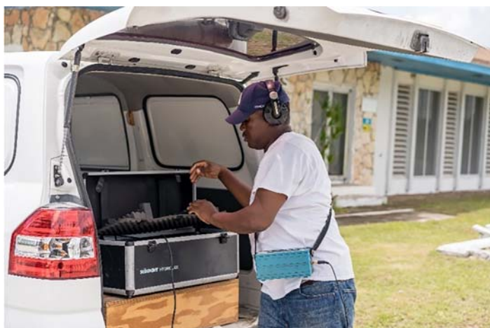
Figure CS2.2 Leak detection in progress (Source: Miya Water).
