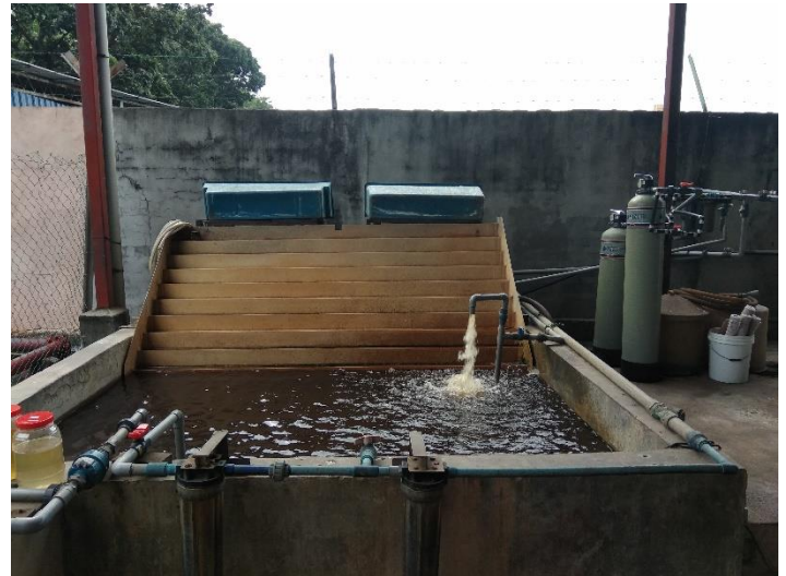
Figure 36: Final Discharge Point
