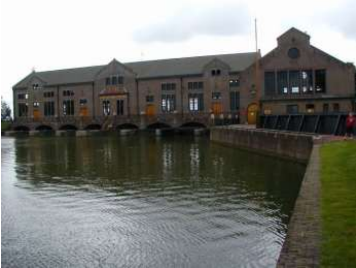
Figure 17.12 The Wouda pumping station was built to drain large areas in Friesland, Netherlands and is the largest steam pumping station ever built. It is now on the World Heritage List.
