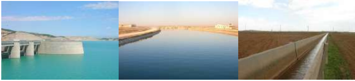
Figure 17.2. The Ataturk dam in Turkey diverts water from the Euphrates River (left). Main canal (middle) conveys water to the Harran Plain for furrow irrigation (right).
