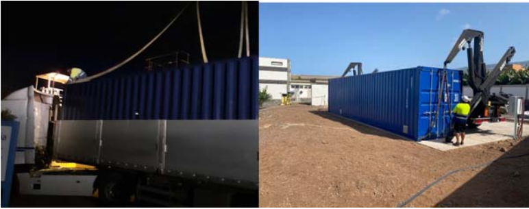
Figure 5.32 Placing the 40-ft. MDC pilot plant containers at (left) the Racons Brackish Water Desalination Plant (Denia) and (right) Demo Site 2 located at Fonsalía Seawater Desalination Plant (Tenerife). Source: Author's own work/property.
