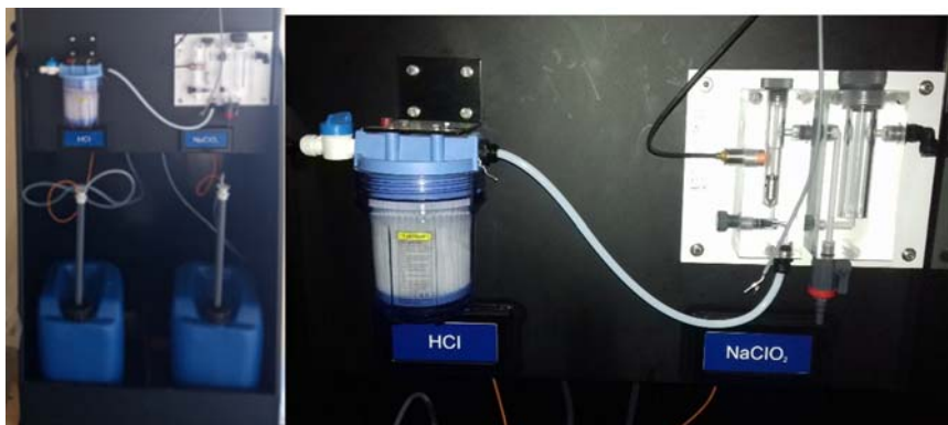
Figure 5.14 \text{ClO}_2 disinfection dosing systems. Source: Author's own work/property.
