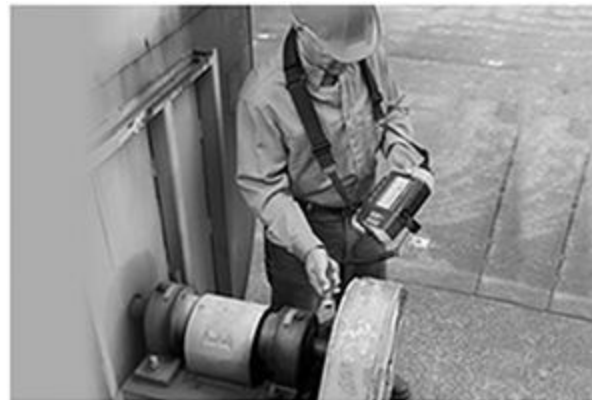
Figure 3.5—Technician Using Vibration Meter with an Accelerometer
