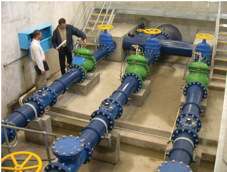
Figure 10.7 Internal view of a portion of the 1065 mm diameter chamber.
