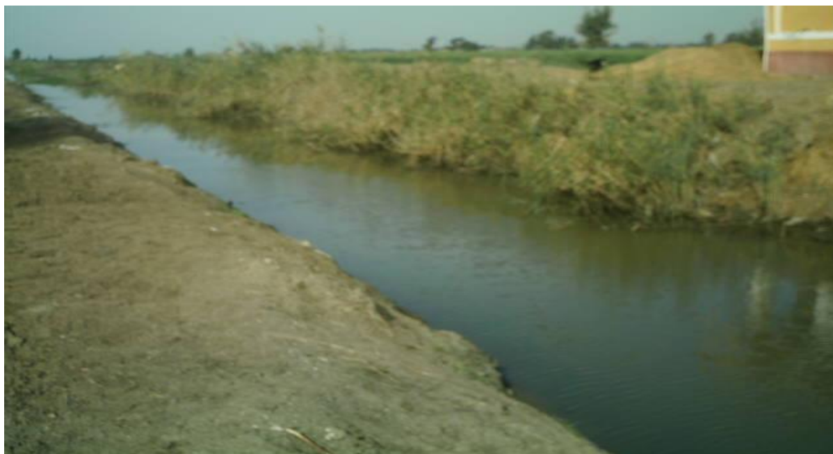
Main Canal in the village
