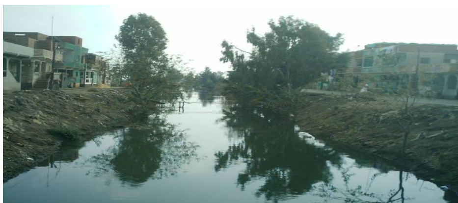
Main canal in the village
