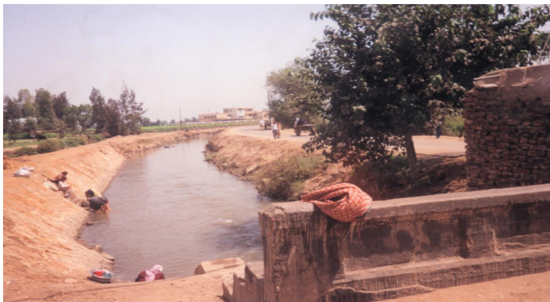
Main canal in the village
