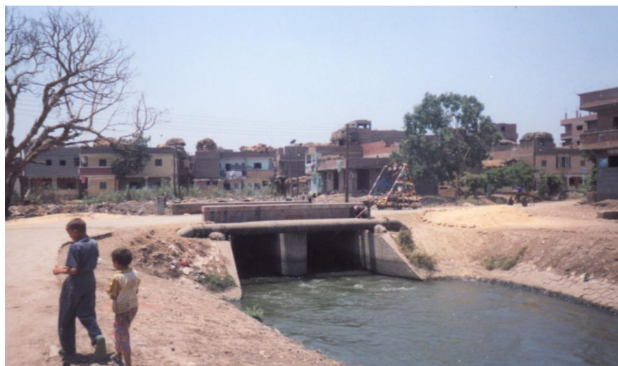
Main canal in the village
