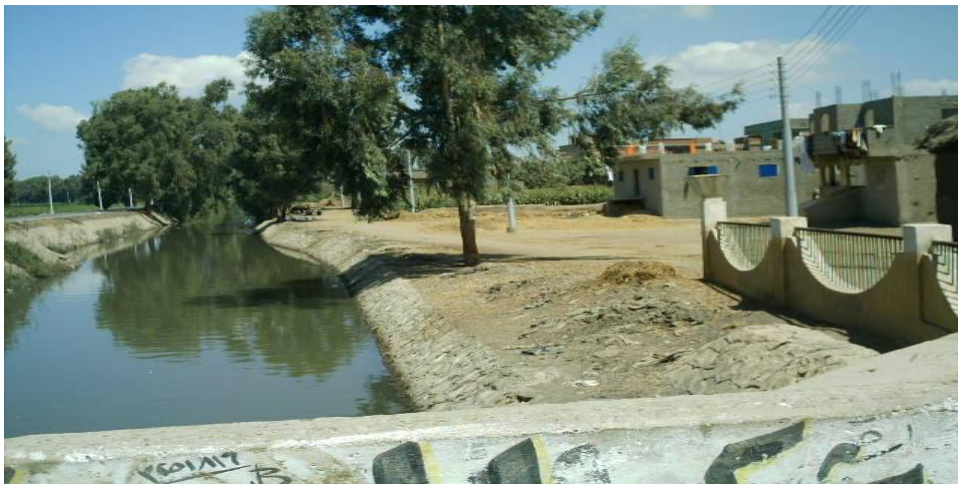
Main Drain in the Village
