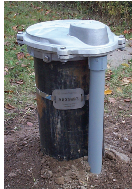
Photo courtesy of Simon Smith Drilling Ltd.
