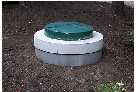
Photo courtesy of Simon Smith Drilling Ltd.
