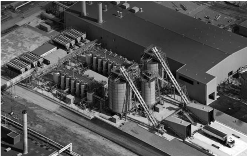
Figure 6.3 Thermal hydrolysis installation at Davyhulme, UK (courtesy: Cambi).
