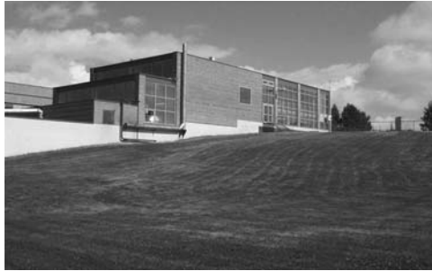
Figure 1.6 Thermal hydrolysis facility in Hias, Norway (Photo courtesy of Cambi).
