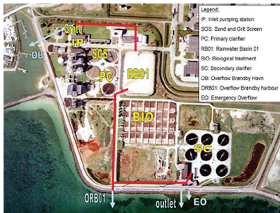
Figure 6.24: Aerial view of Avedøre WWTP.
