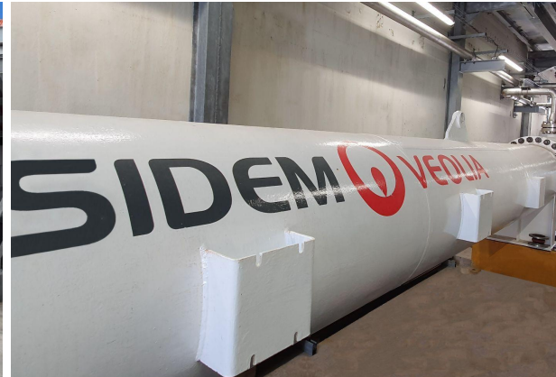
St Barthelemy - SWRO BARREL™ B1 - 1 x 800 m 3 /d unit
