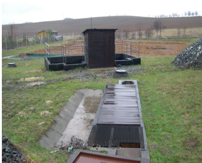
Figure 3.5 Ondřejov HF wetland: sand trap (front), Imhof tank and vegetated HF bed (back). Photo courtesy of Jan Vymazal.
