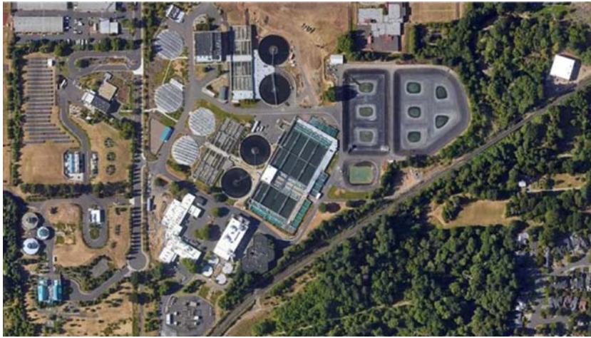
Figure 6.1 Durham advanced wastewater treatment facility.
