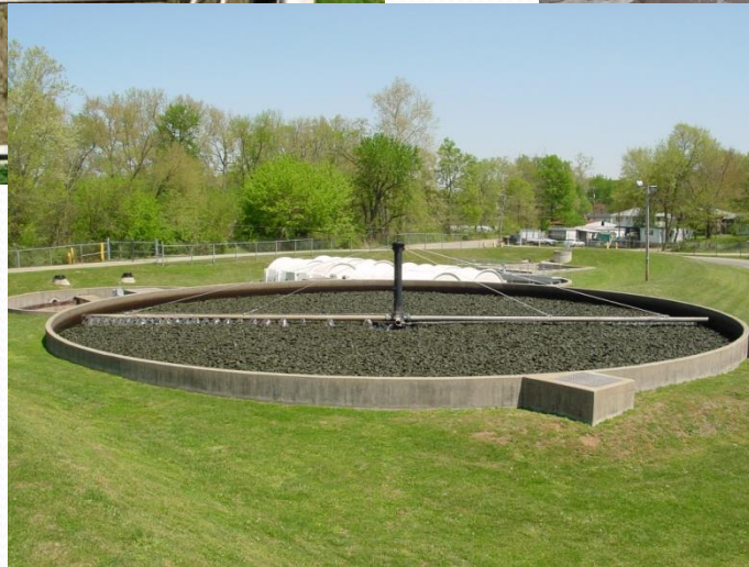
Trickling Filter
