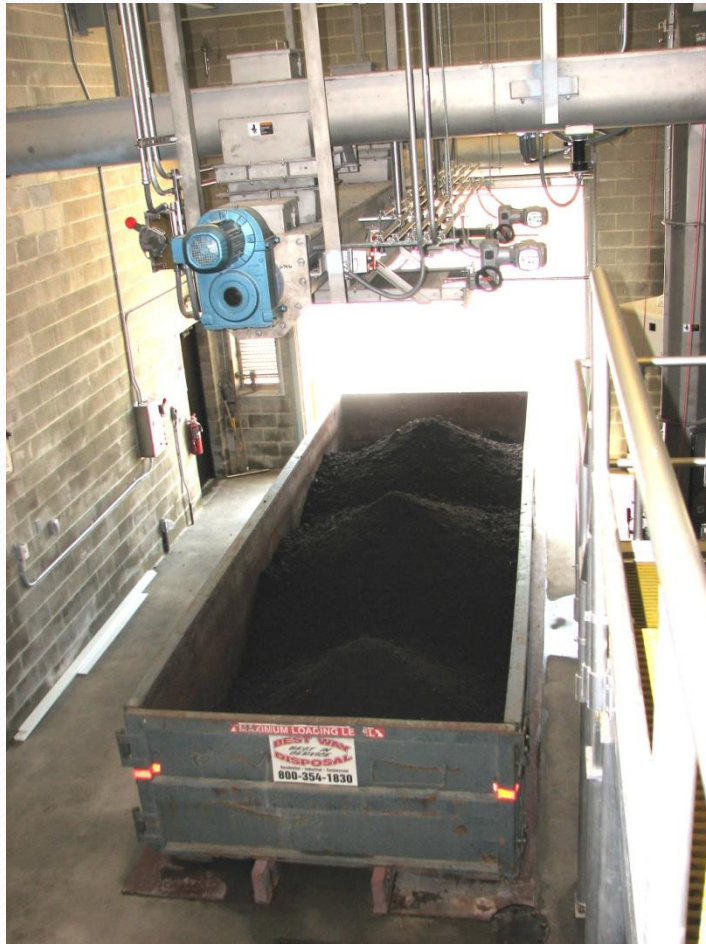
Dewatered Sludge from Belt Presses to Landfill
