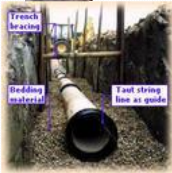
Laying New Sewer Pipes
