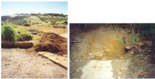
Visual inspection of site soil erosion & drainage management measures and a discharge point
