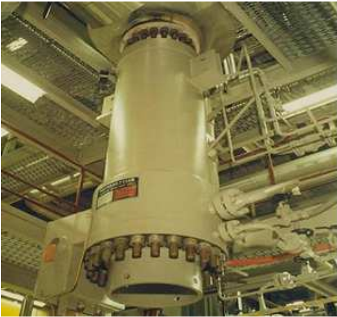
Photograph 14: Typical BWCP (Boiler Water Circulating Pump) Installation
