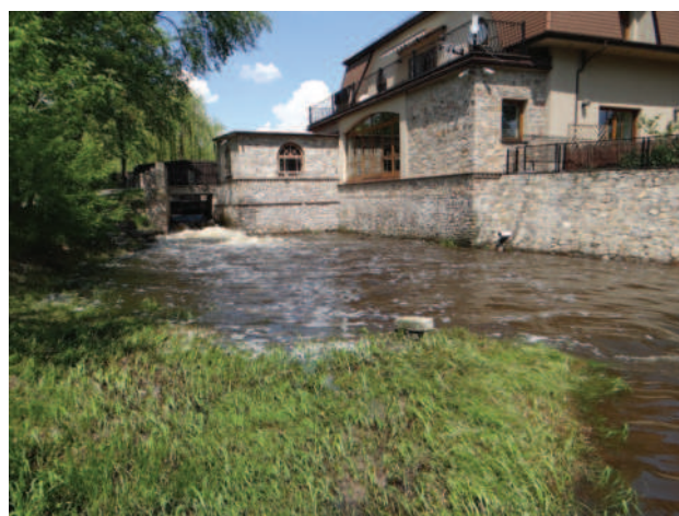
Figure 1. Renovated water mill before transformation into SHP
