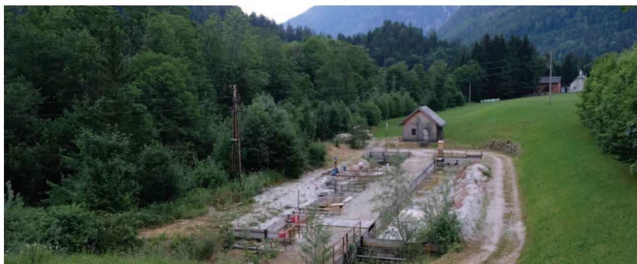
Figure 4. Research facility hydromorphological and temperature experiment channel
