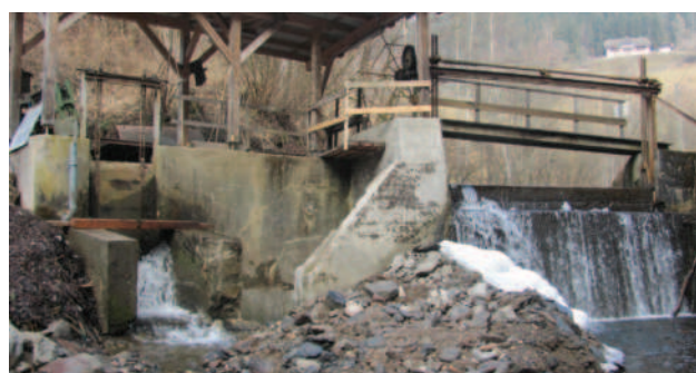
Figure 2. Pilot plant Löllingbach
