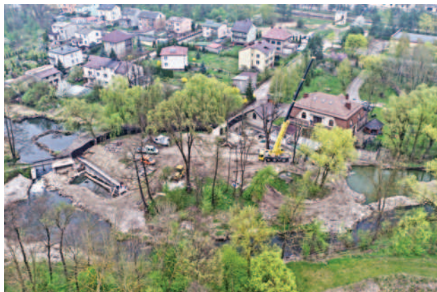
Figure 4. Construction area during the installation of the Archimedes' screw. The old hydro-technological system supplemented with the newly built fish pass is visible
