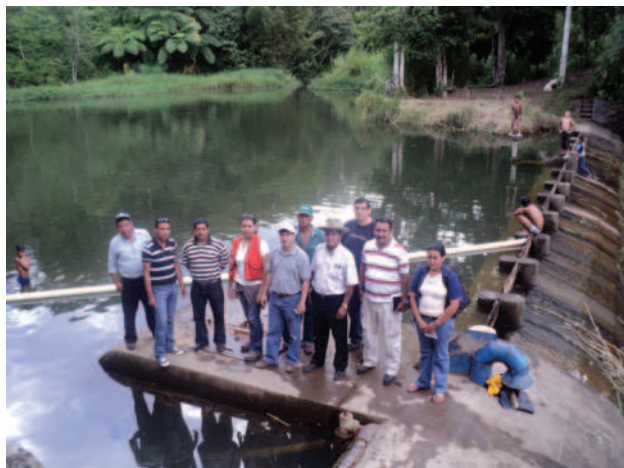
Figure 5. Dam of the El Bote hydropower plant
