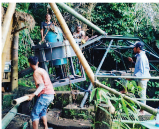
Figure 9. Bamboo crane, Green School, Bali Indonesia
