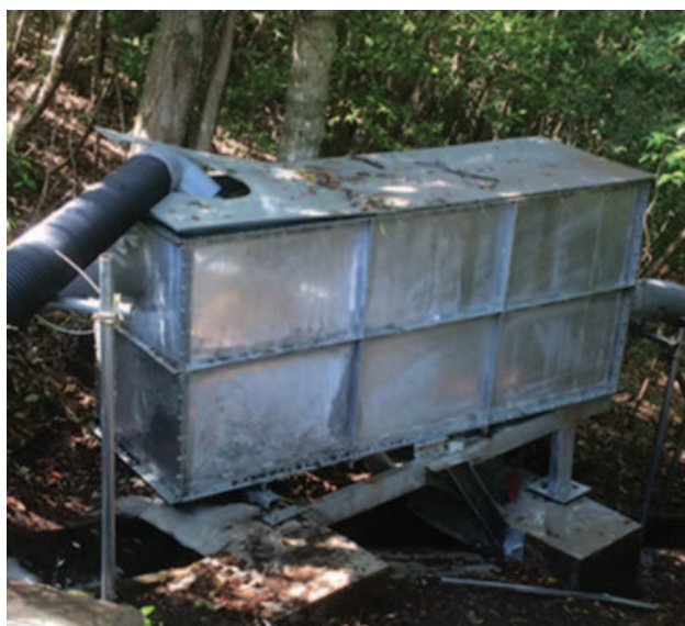
Figure 1. The head tank from the intake
