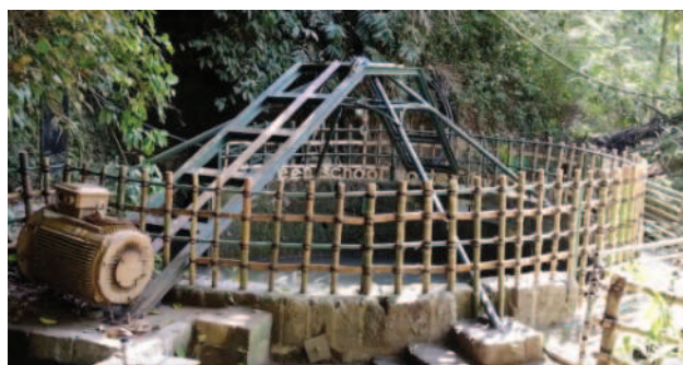
Figure 5. Green School's self-made bamboo security fence
