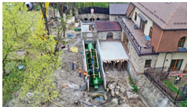
Figure 2. A challenge during the installation of the Archimedes' screw was its transportation from the semi-trailer to the channel because of high trees located in the immediate neighbourhood
