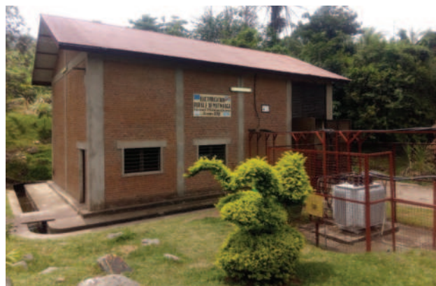
Figure 3. The powerhouse of the Mutwanga SHP
