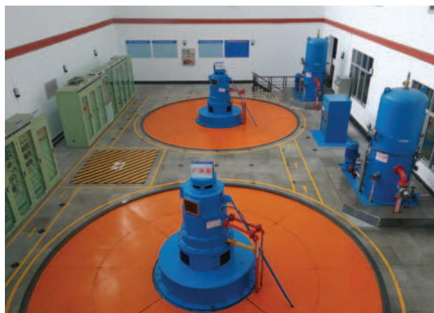
Figure 1. The powerhouse of the Mantianting SHP
