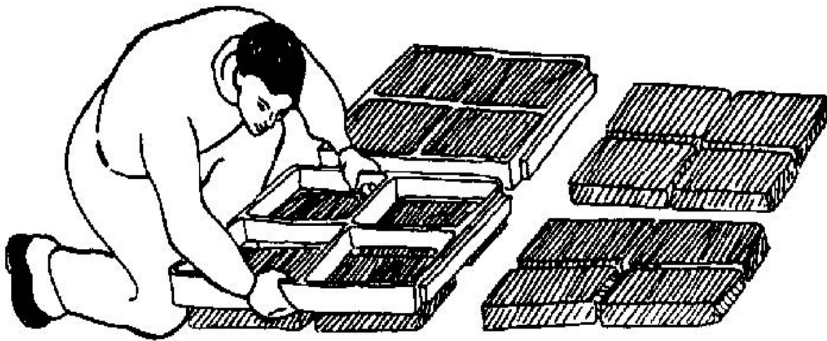
Figure 41. Lifting the forms from freshly made blocks.
