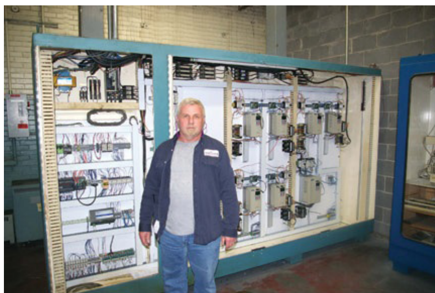
Figure 3: Jonathan Payton stands in front of the new finishing line control cabinet which includes a DL260 DirectLogic PLC, 8 Durapulse variable frequency drives, and all the associated control equipment. The entire design including software was installed during their 3-week shutdown.
