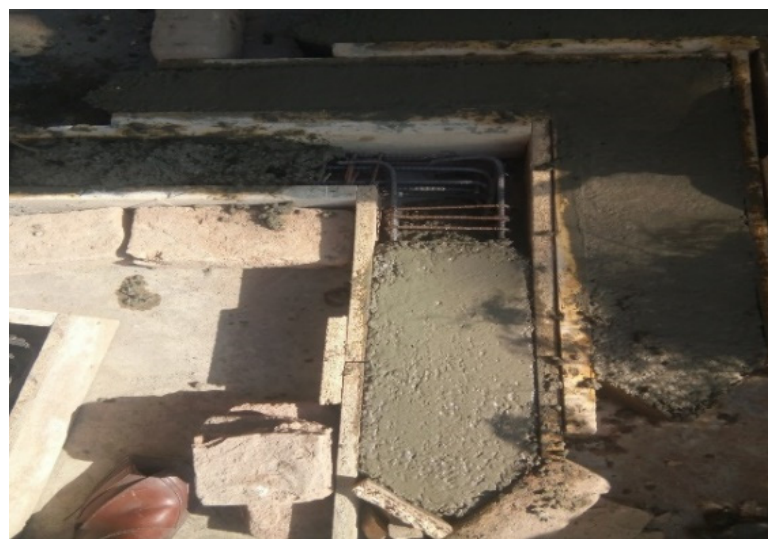
Figure 3. Joint left for RPC.
