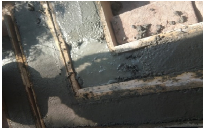
Figure 4. Joint filled with RPC concrete.
