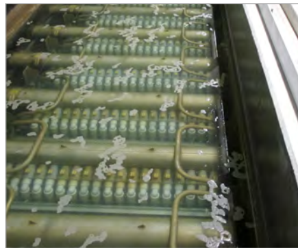
Figure 4: Membrane Bioreactor (MBR)
