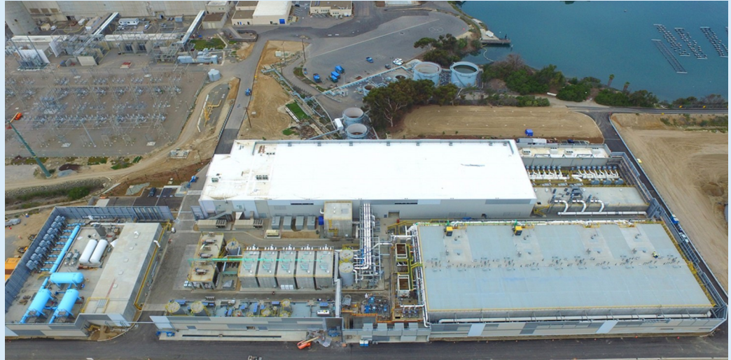
San Diego Water Authority Claude "Bud" Lewis Carlsbad Desalination Plant, Carlsbad, CA
