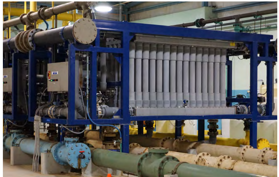
Figure 4: Example of encased (pressure) membranes
