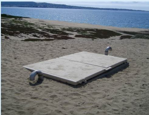
Seawater desalination facilities in California are employing beach wells to reduce pretreatment requirements and improve plant efficiency.
