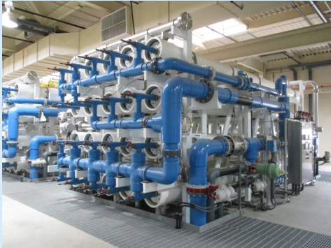
Innovations in membrane design, such as this 16-inch configuration at a potable reuse facility, are creating more efficient designs and lower treatment costs.
