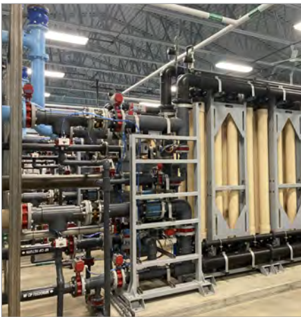
Figure 3: Microfiltration/Ultrafiltration
