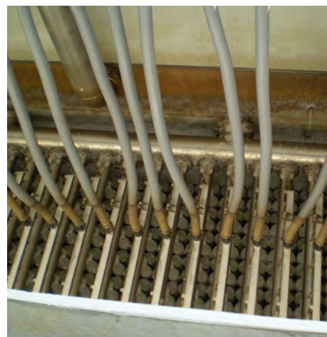
Figure 5: Example of immersed (submerged) membranes
