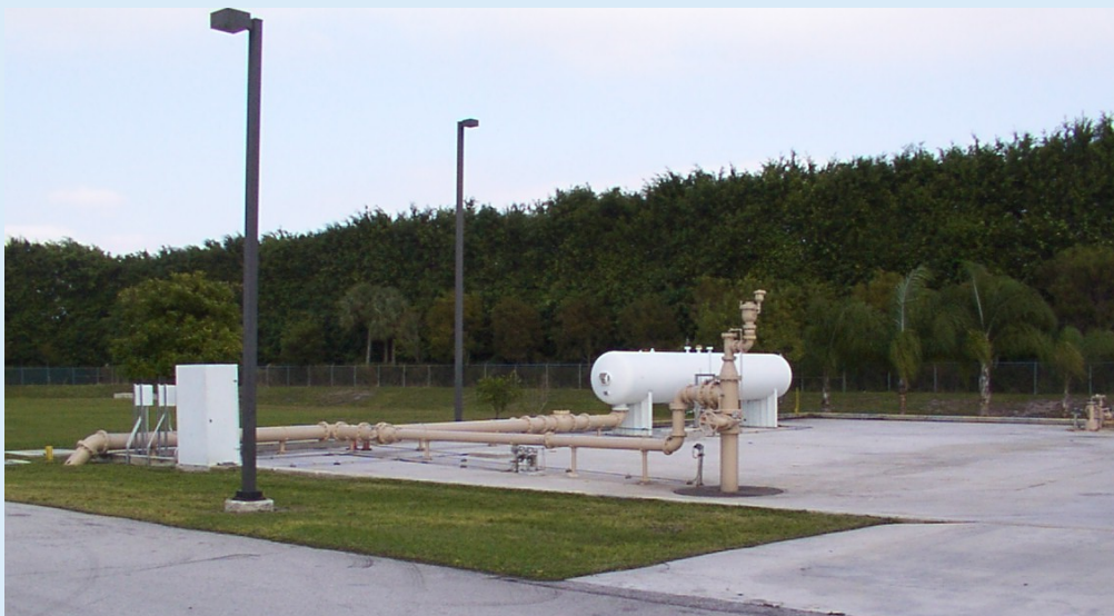
Injection wells can be used for disposal of concentrate
