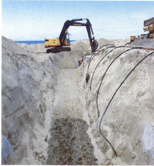
Figure G.1: Construction of coastal drains
