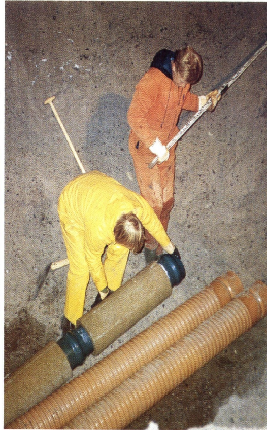
Figure G.1: Construction of coastal drains
