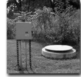
Submersible lift stations are designed to blend readily with natural surroundings, since there is no pump house and there is a minimum of above-ground equipment. Discharge to below-ground installations are holes and use safety-hazard concerns.
