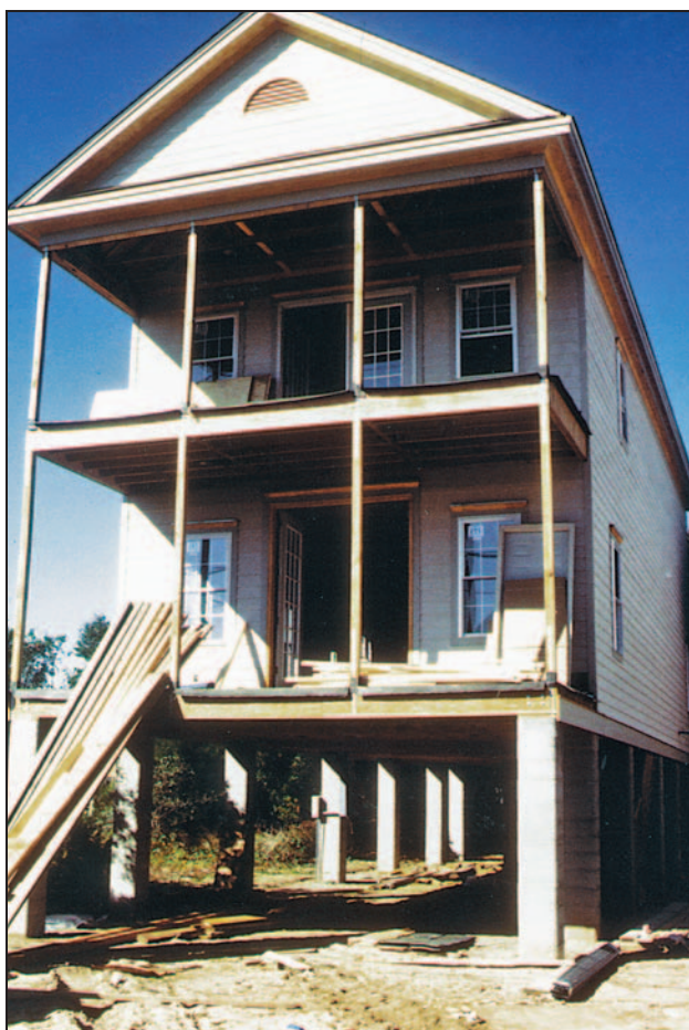
Figure 13-6. Open masonry foundation
