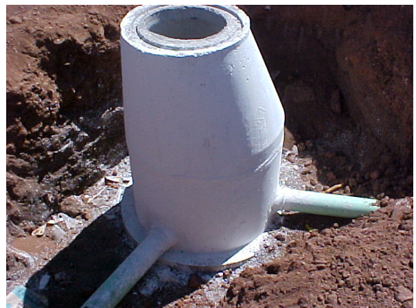
Newly finished Manhole and Laterals.
