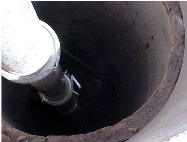
Looking down inside the manhole.
