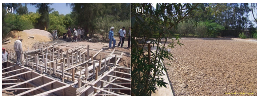
Fig. 5.8 (a) Construction of the septic tank, (b) Constructed wetlands before planting in Sharquiya
