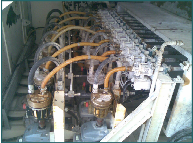
➤ MIXING & PUMPING PROCESS
