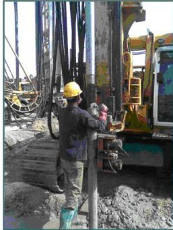
EXCEEDING PIPE LENGTH TO REACH TO THE FINAL DEPTH
