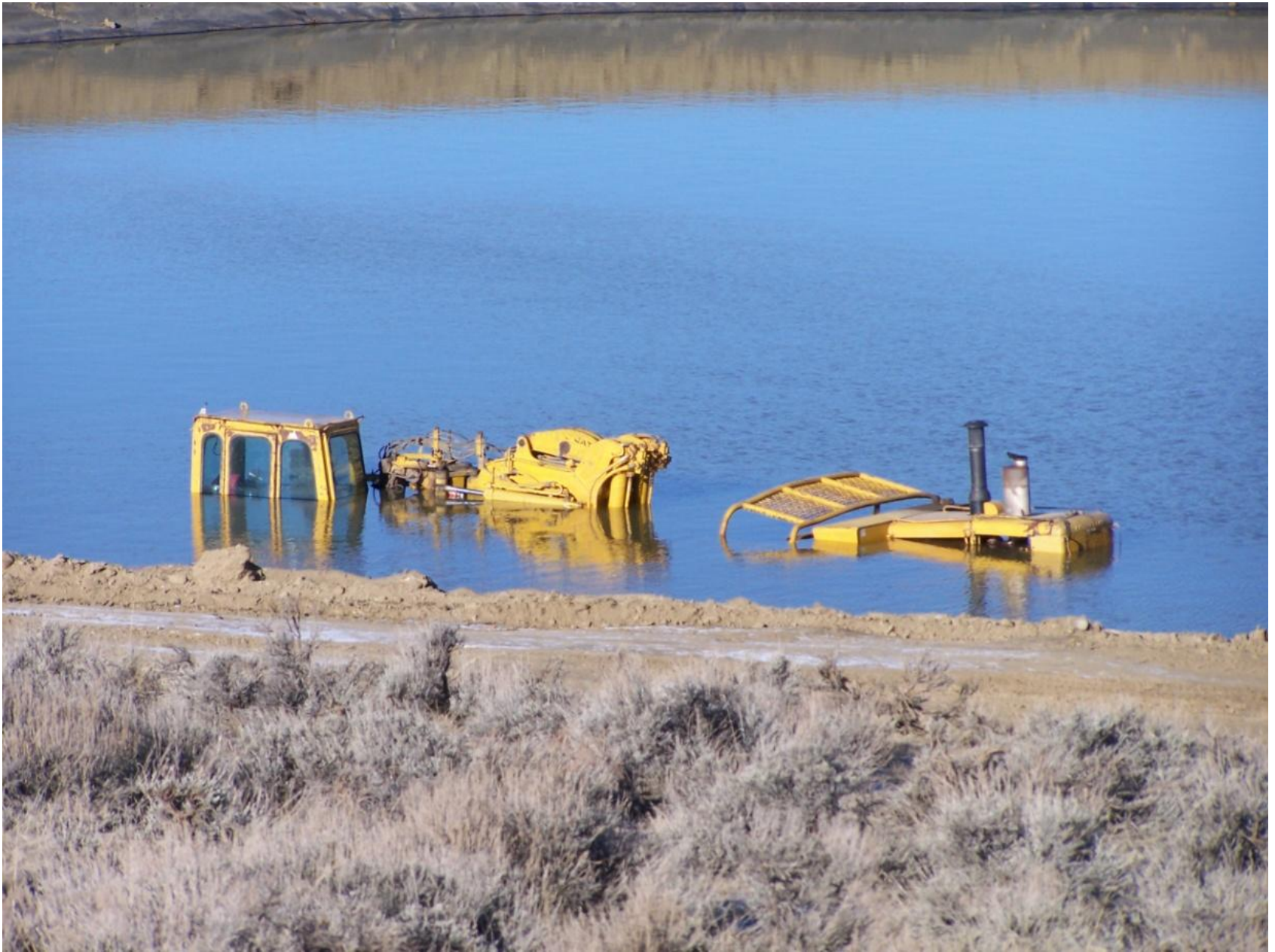
Picture 10 - Hazard Potential
