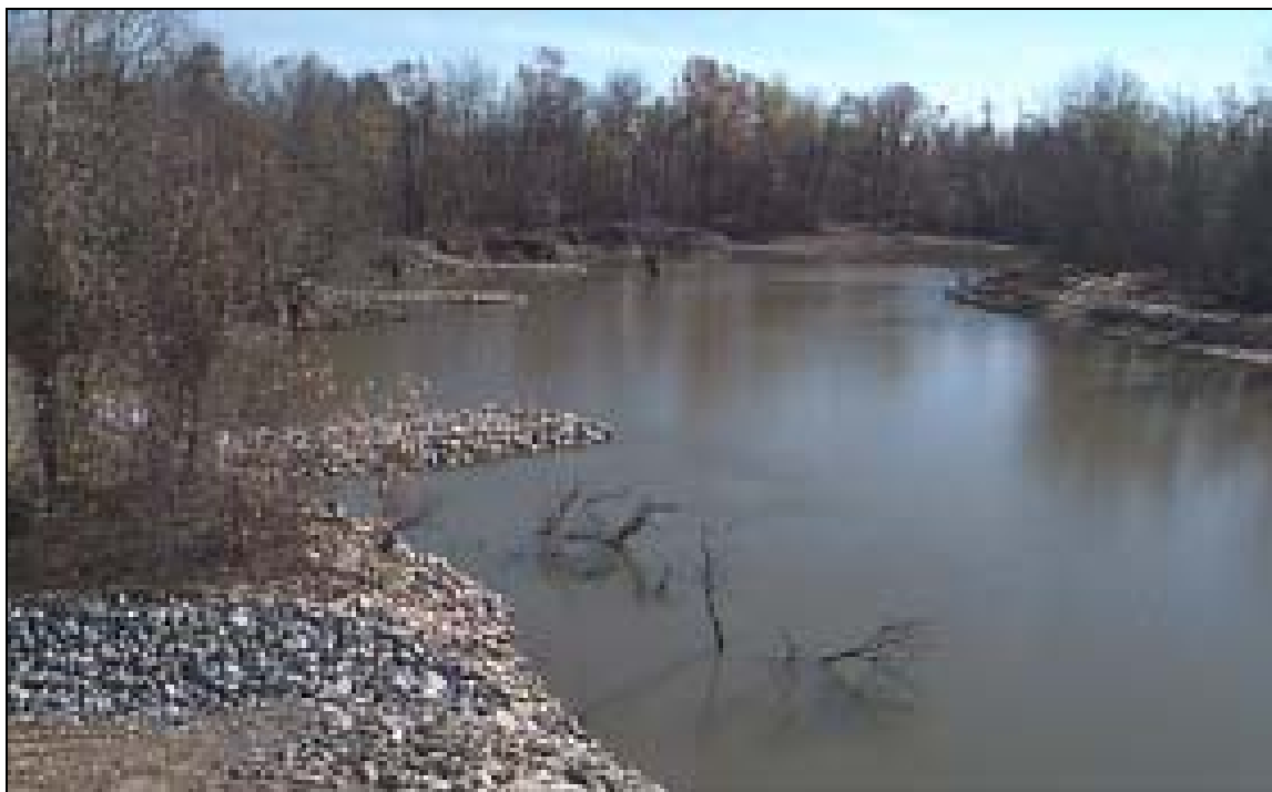
Figure 5.41. Bendway wiers on outer bank of Hatchie River looking upstream (TDOT).
