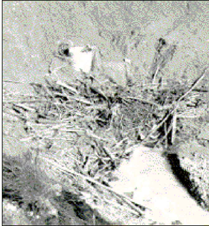
Figure 5.25. Installation shown in Figure 5.24 after flood. Riser conveyed large flows during flood. Fence partially surrounding riser was of no value for debris control.
