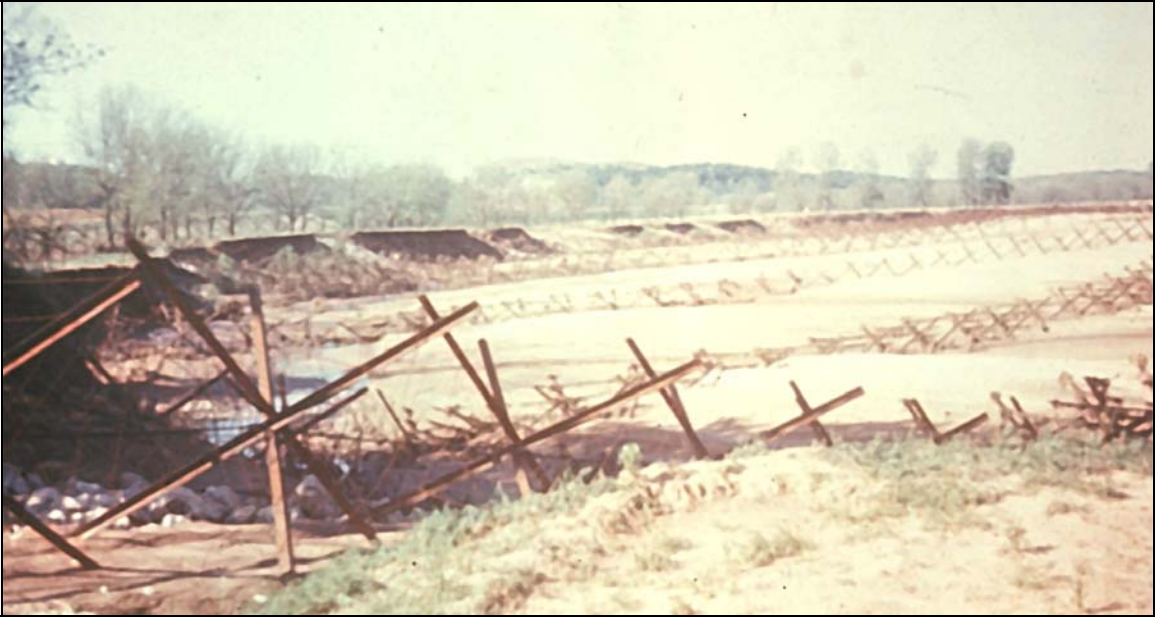
Figure 5.42. Kellner jacks used for redirecting the flow patterns.
