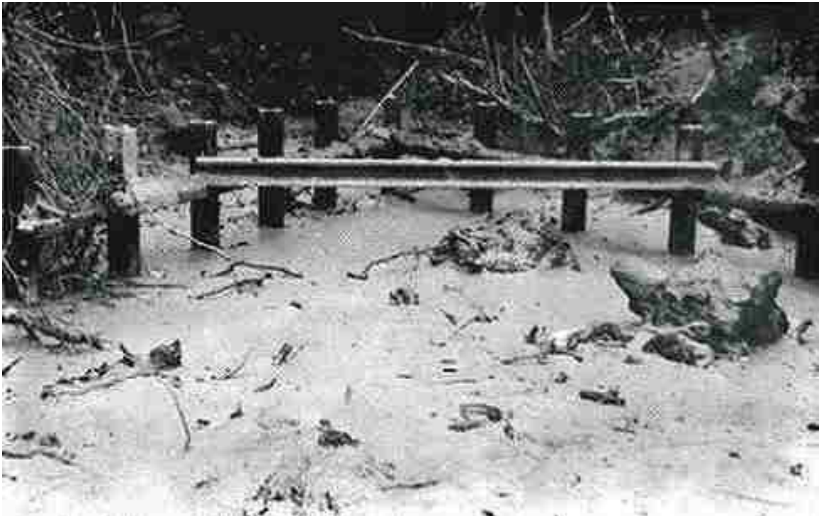
Figure 5.7. Steel rail debris deflector in area of heavy flowing debris (looking upstream).
