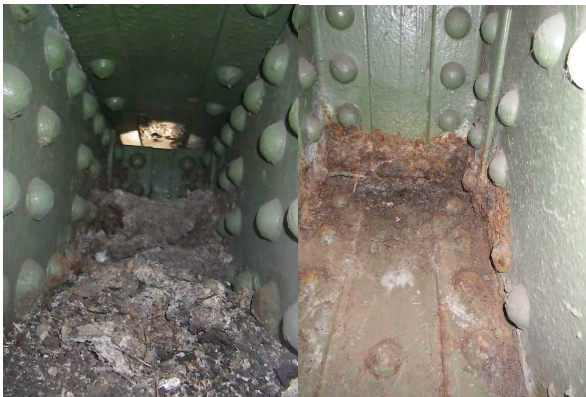
Figure 2. Bottom chord interiors
