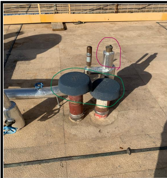
Drainage Vent Cap , Water Supply and Fire Fighting Automatic Air Vent Site Installation
