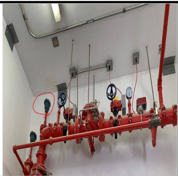
Drainage Vent Cap , Water Supply and Fire Fighting Automatic Air Vent Site Installation
