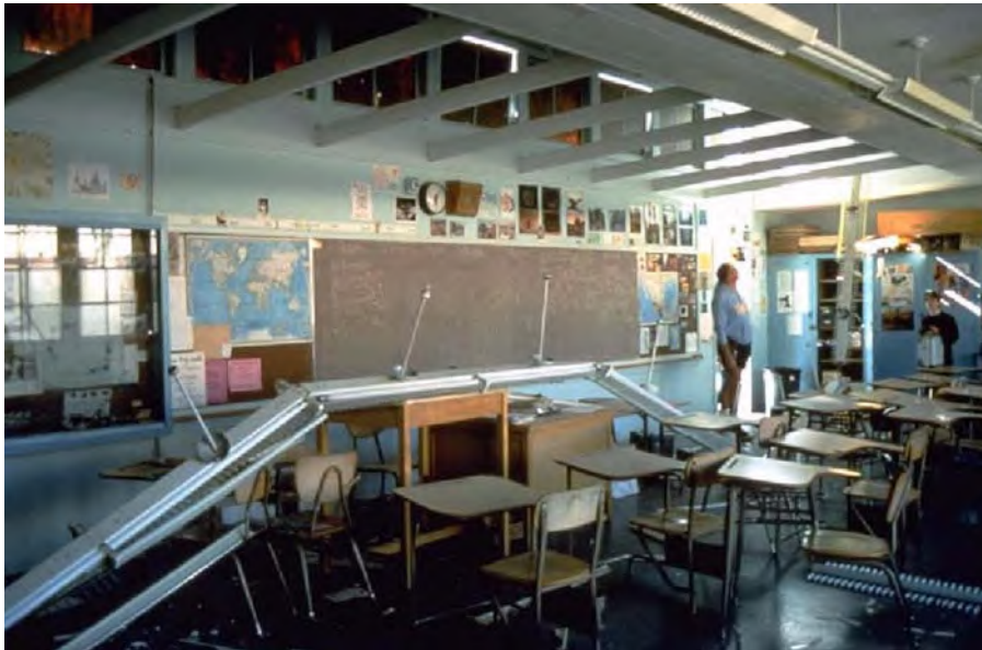
Figure 10-1 Nonstructural damage at Northridge Junior High where lights fell onto desks during the 1994 Northridge earthquake. (photo courtesy of the Earthquake Engineering Research Institute)
