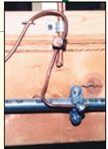
Install bonding jumpers around nonconductive material.
